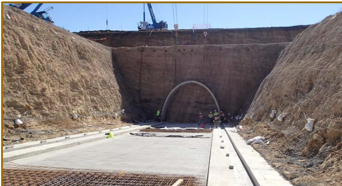
*First portal arch installed in the box cut at Eagle Downs*
