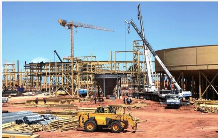
Erection of steelwork for process plant
