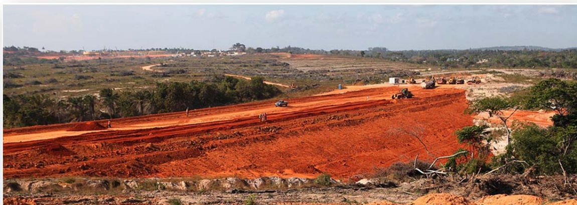
Tailings dam embankment
