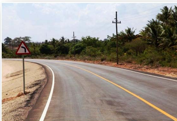
Mine access road essentially complete
