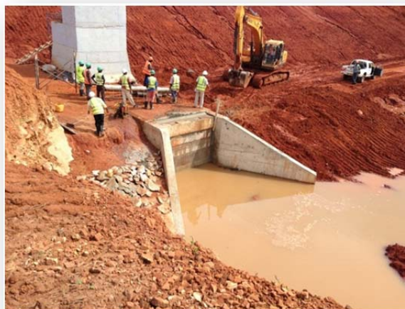
River diversion channel with plug in place
