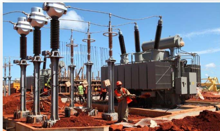
Construction of the mine substation
