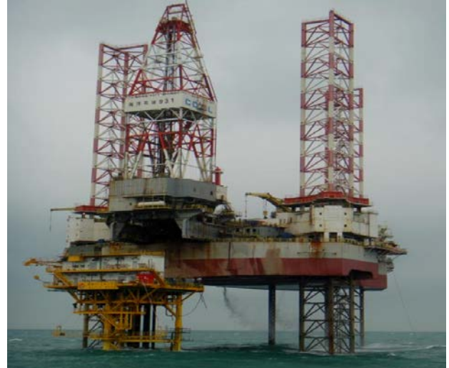
Figure 2: COSL HYSY 931 Rig at WZ6-12 WHP Platform for Development Operations
