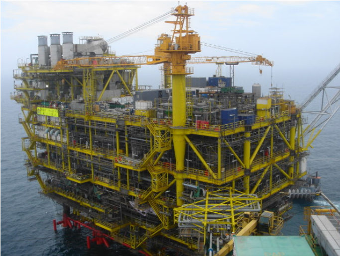
Figure 1: Newly Installed PUQB Processing Platform
