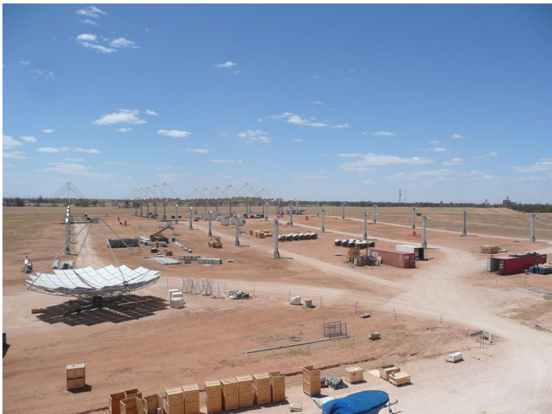
Plant construction at Mildura, Victoria - February 2013
