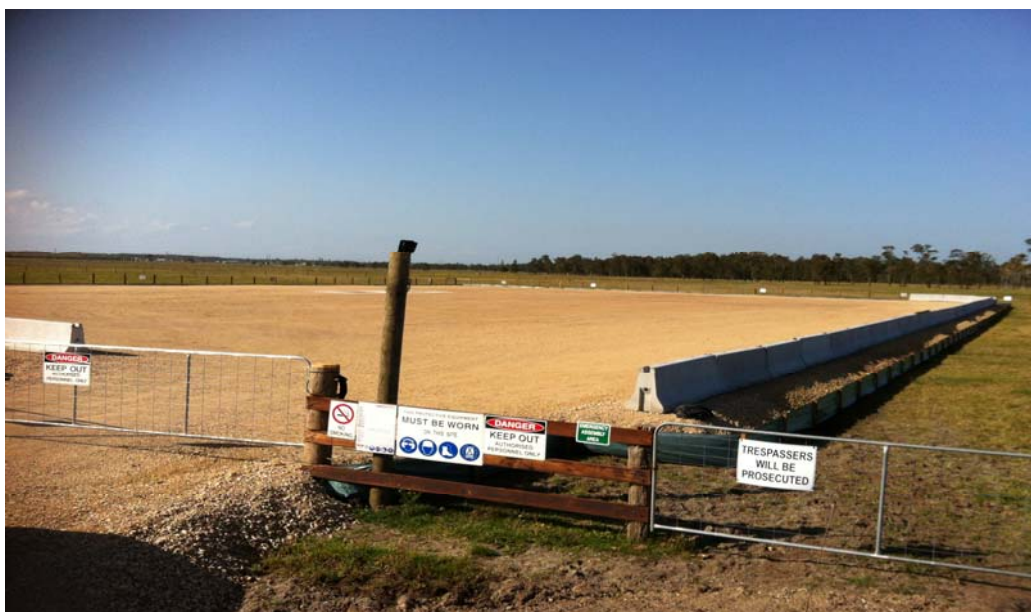
Fullerton Cove drill site, New South Wales
