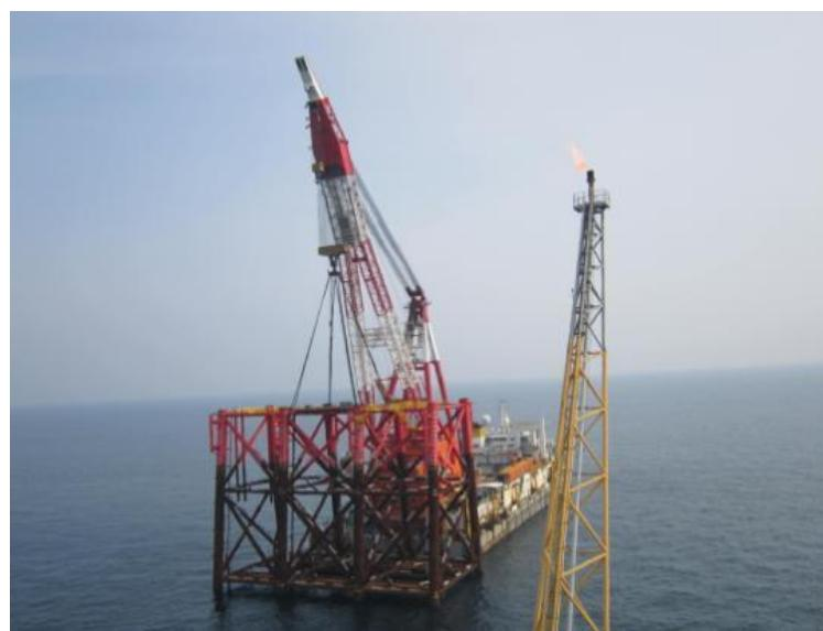
PUQB jacket lift by heavy lift vessel Lanjiang near CNOOC WZ 12-I production complex
