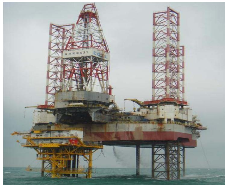
COSL HYSY 931 jack-up rig drilling over WZ 6-12 wellhead platform
