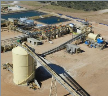
Crushed ore bin and flotation circuit
